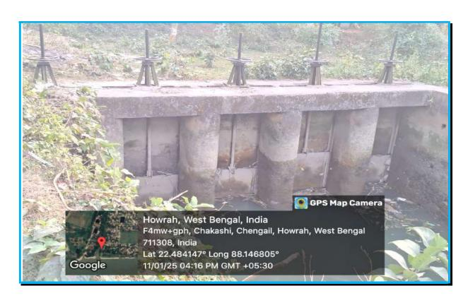
**Name of Project:-** Replacement of 5 nos Flap Shutter including guide path, bottom seal, painting, hoisting arrangement and Cross bandth at **Gouriganga**, Block -Uluberia Municipality, P.S- Uluberia, Dist. Howrah.
