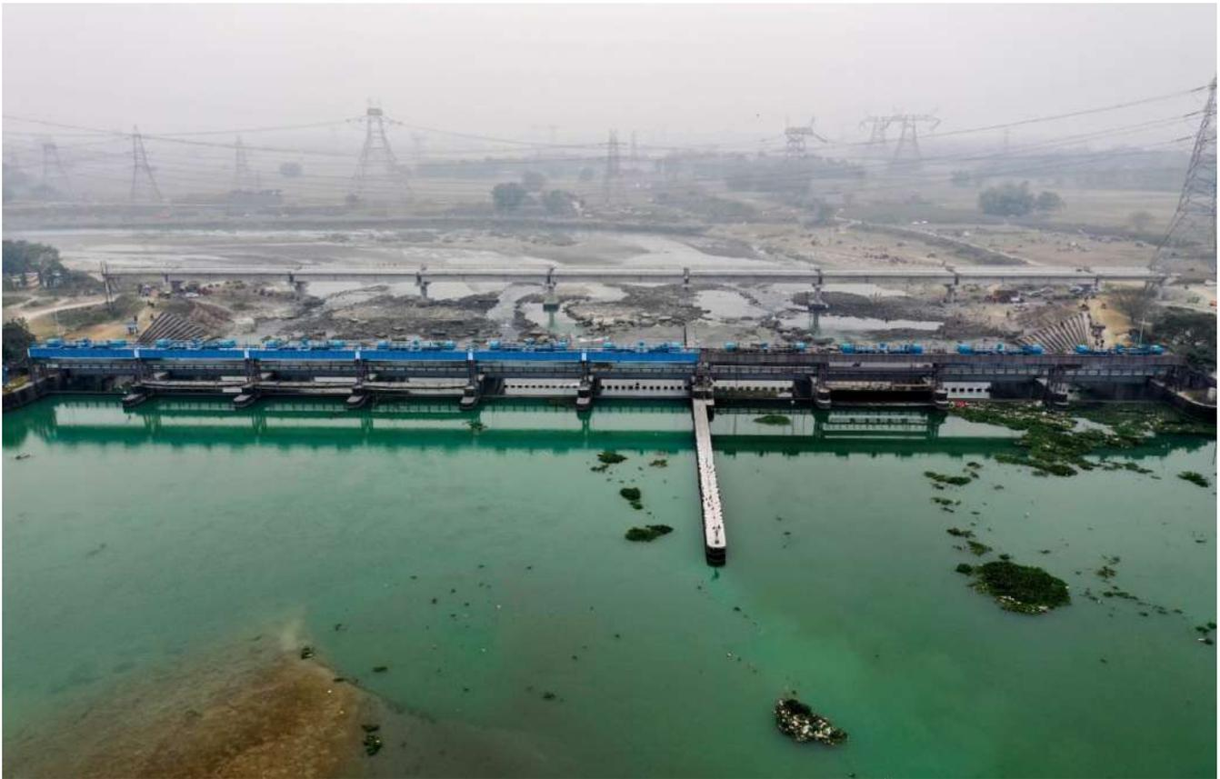
Fig 1: Mahananda Barrage and Head Regulators on right bank.
