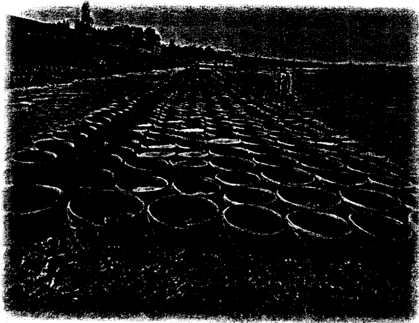
Teracotta rings may be used as silt trapping unit
