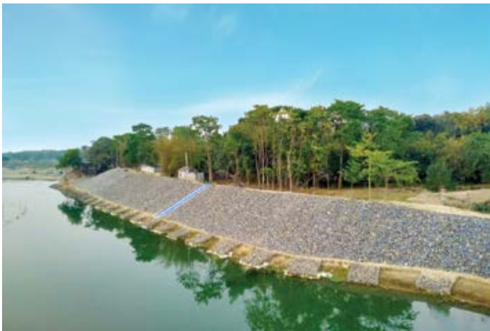
Figure 6 Bank protection work on river Teesta at Padomoti in Jalpaiguri district
