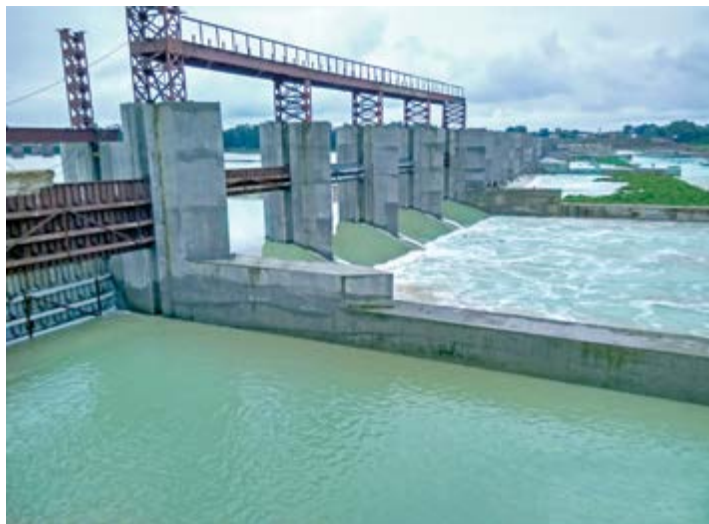
Figure 1 Reconstructed Anicut structure over Kangsabati River at Mohanpur
