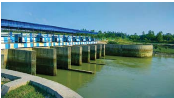
Figure 4 10-vent Sluice structure in Sagar Block of South 24 Parganas
