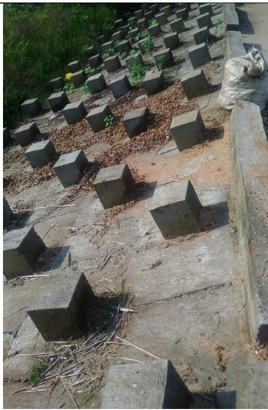
Figure 56: Wave breaker (country side) provided on spill zone located on Damodar Right Embankment at Shibani para
