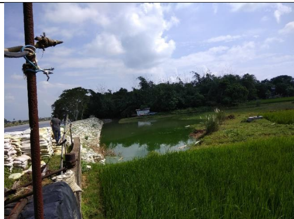
Figure 53: Ring band protection with Gunny bag at breach point (during 2017) of Damodar Right Embankment near Tokapur River Lift point
