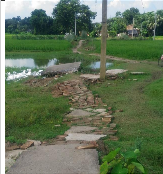
Figure 57: Breach point (2017) of Damodar Right dwarf embankment located near Tokapur River Lift point
