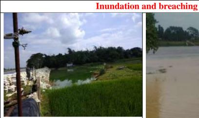
Figure 53: Ring band protection with Gunny bag at breach point (during 2017) of Damodar Right Embankment near Tokapur River Lift point
